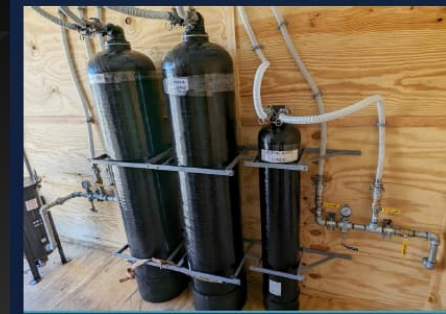
PFAS IDW Treatment System Pilot System Vessels
