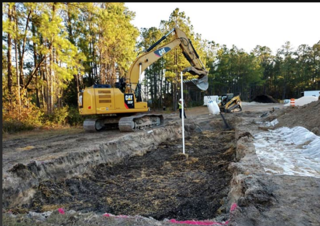
SBGR Construction – Mixing Amendments into Reactive Media
