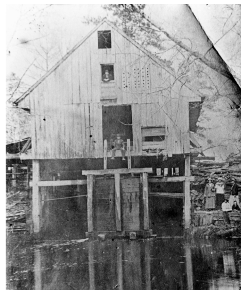
Early twentieth century image of Henderson's Mill, owned by Isaac Newton Henderson. The water-powered saw- and grist mill was located on Queens Creek.
