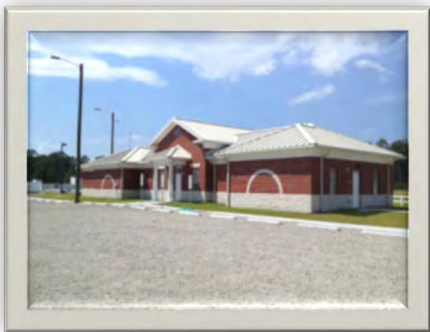
Clubhouse and Retail Facility
