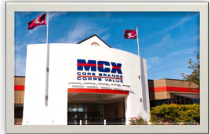
Main Exchange Entrance
